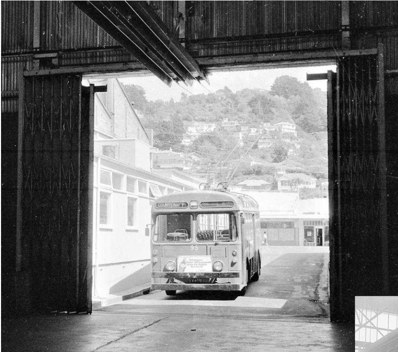
Left: 95 waits in the sunshine outside the depot. Most of these nineteen B.U.T.s saw an average of twenty-two years service. We must be grateful to Graeme Bennett for recording these scenes which were later swept away when part of the depot land was sold and a retirement village built in its place.
