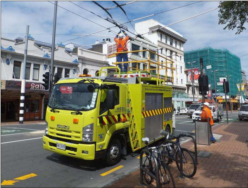
Left: Tower wagon TS1, a 2014 Isuzu FRR, was photographed in Courtenay Place with staff working on the switch at the eastern end that separated the routes taking trolleybuses through Hataitai (left) or Newtown (straight ahead).
