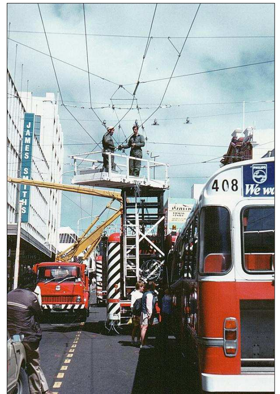
Below: A view further along Cuba Street with 1983 Bedford cherry picker 961 at the kerbside. Photos: NZ Bus collection.
